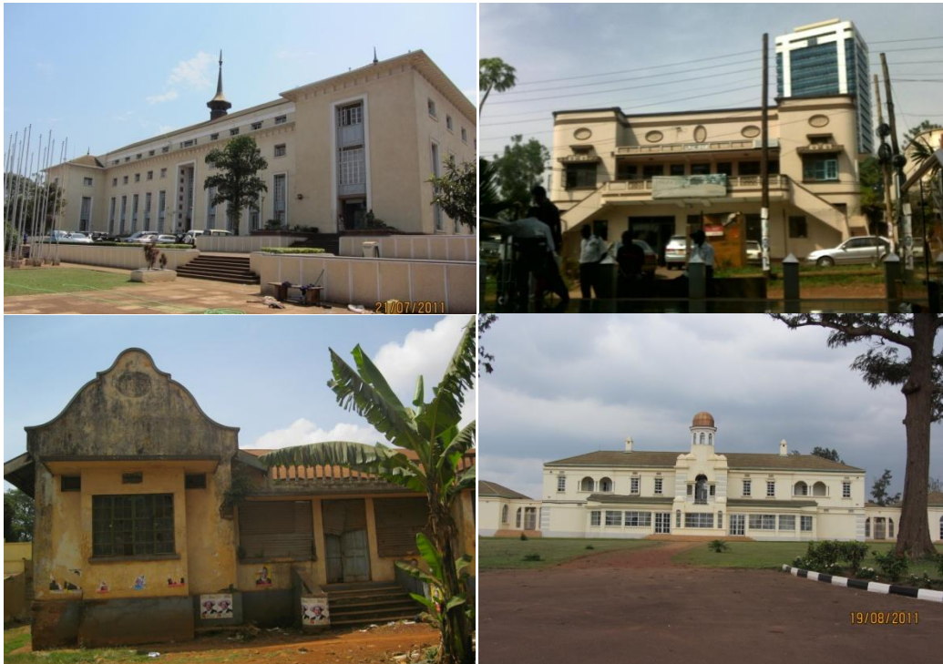
Figure 25: Examples of Historic Buildings, Kampala, 2011
