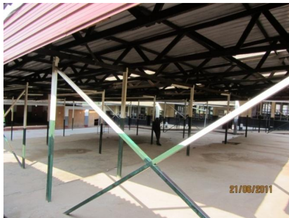
Figure 59: Covered Assembly Ground, Nakasero Primary School
