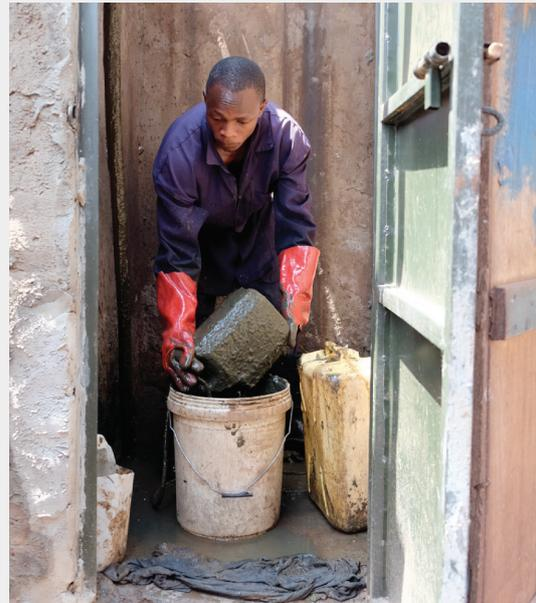
Figure 4: Scooping sludge from a pit latrine
