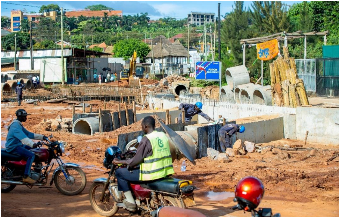
Cape Road Ggaba – Drainage Improvement
