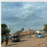
Kinawataka road 1.9km
