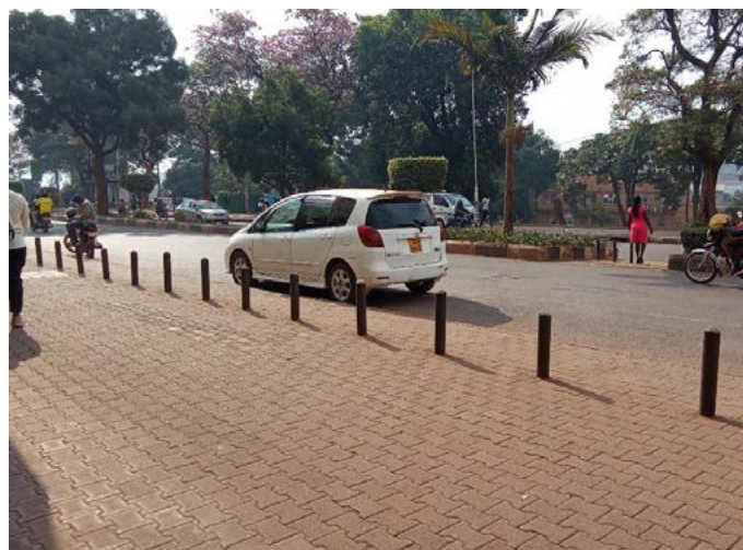
Figure 4.12: Traffic island access for pedestrians at Kampala Road; walkway protected from parking encroachment
