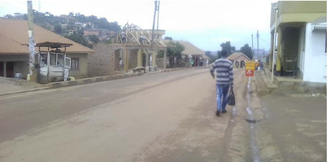
Figure 4.16: Kulekaana road at the junction going to Mirembe primary school (no walkways, pedestrian walking in the carriage way)
