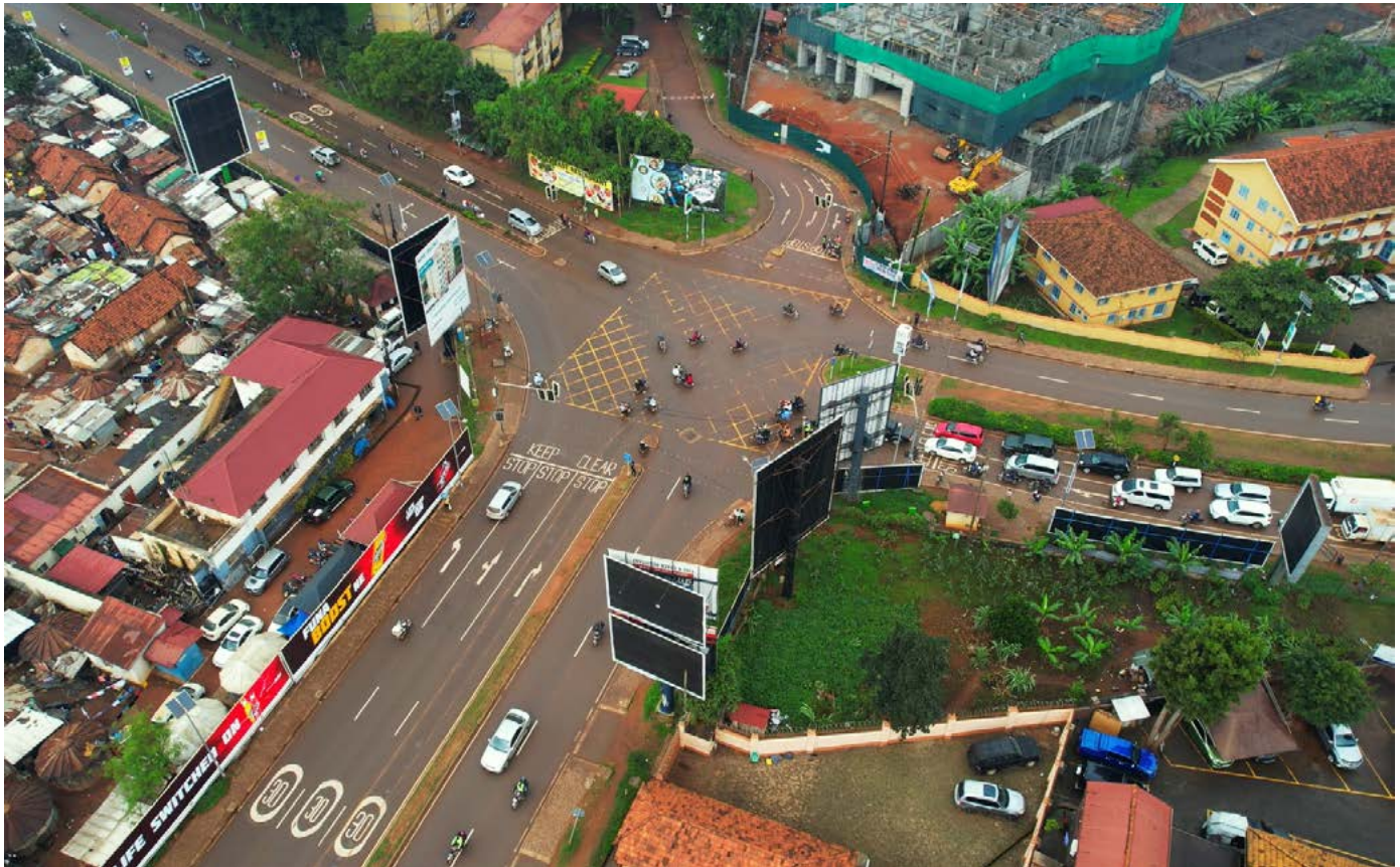
Figure 7.12: Marking of Lane lines, lane direction, speed limit, stop lines and Keep clear at Kira Road- Lugogo Bypass intersection. Source: WRI
