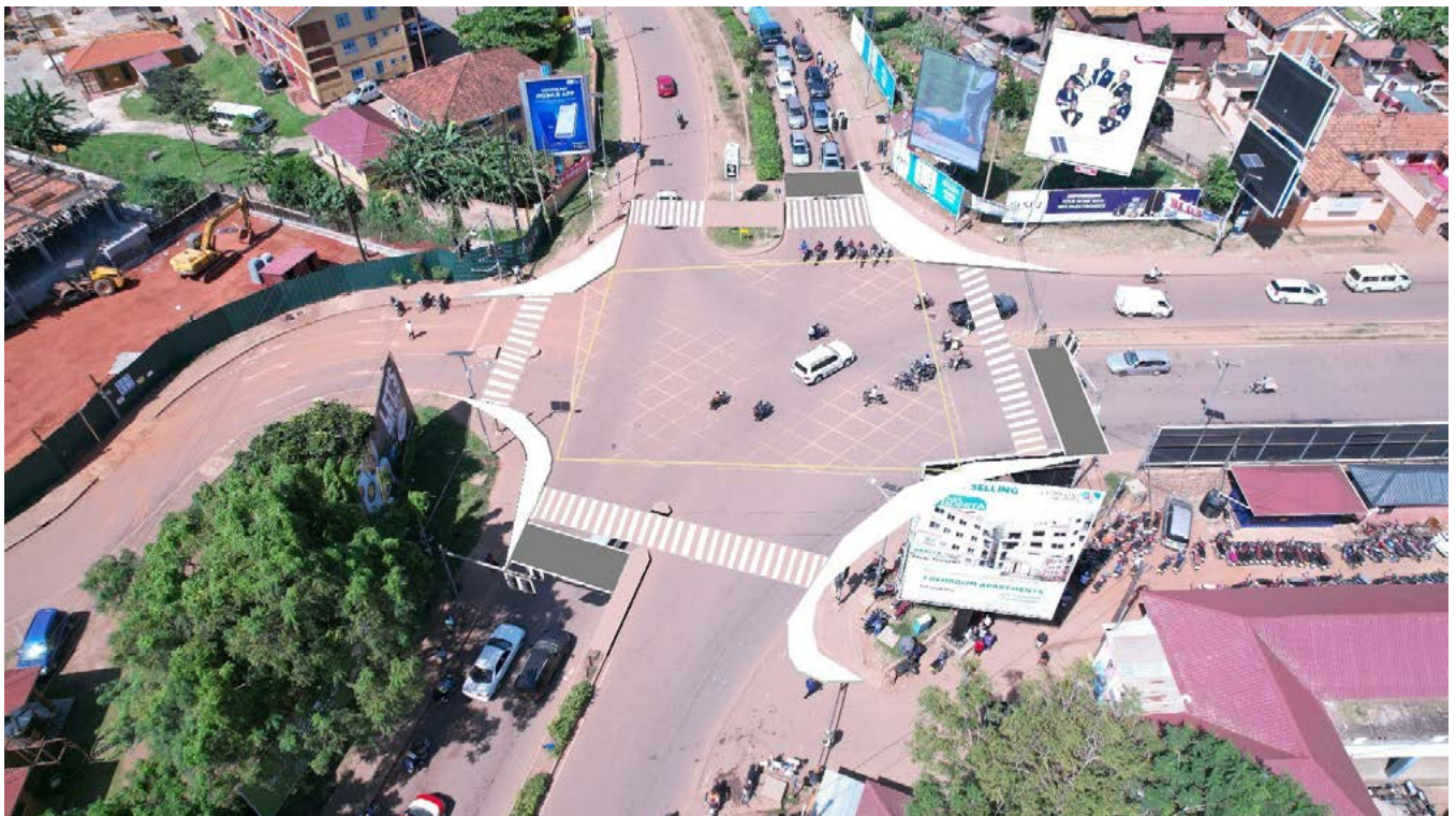
Figure 7.11: Proposed interventions for Kira Road- Lugogo Bypass Intersection- road marking renewal, advanced stop boxes, curb extensions, more direct crossing points.
