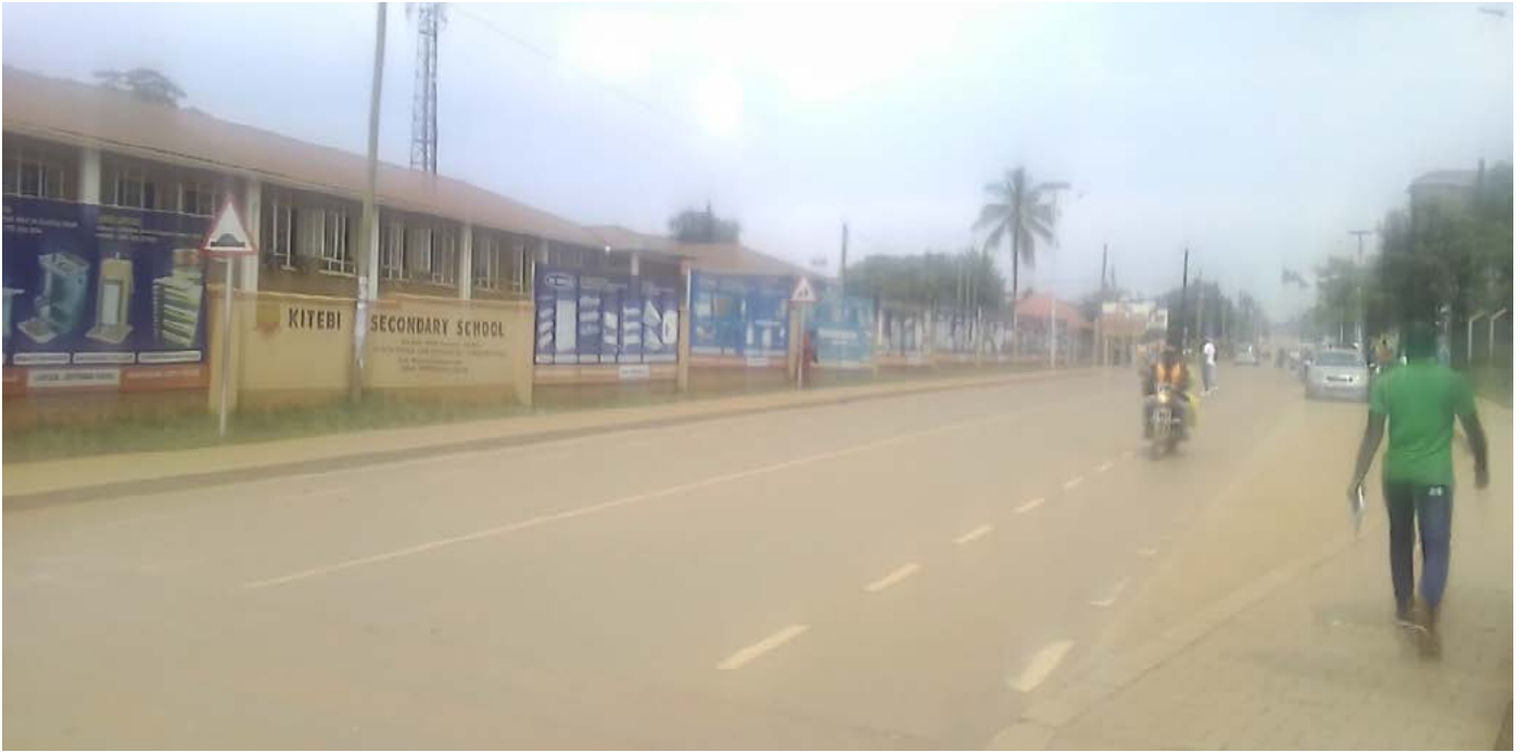
Figure 4.15: Wankulukuku Road at location between Kitebi Primary and Secondary Schools (adequate walkways)
